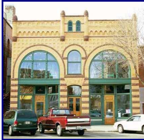
NOHR's Offices The Wagner Building
